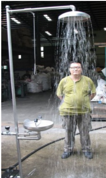
Shower head give a concertrated flow of water in a drench colum with radius of 200mm comply to ANSI/ISEA Z 358.1 : 2014
